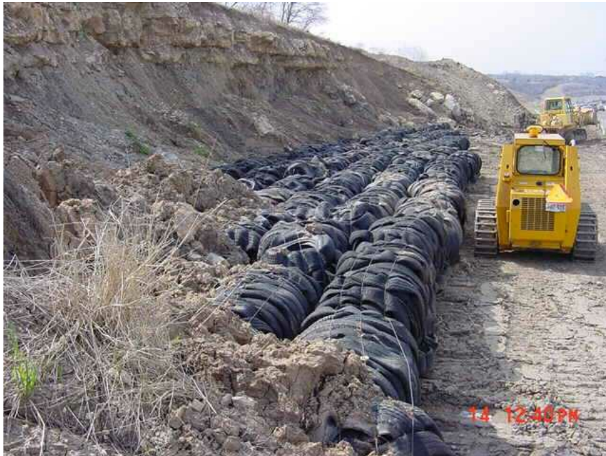
Scrap tire bales placed at toe of slope.
