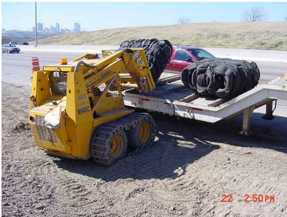
Scrap tire bales can be placed using readily available equipment.
